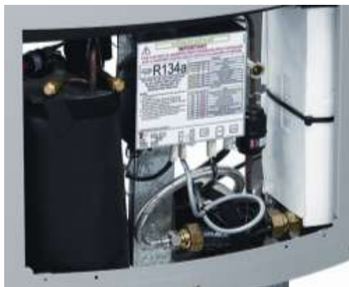
Steps 11 and 13 remove front cover from heat pump module and feed through cables
