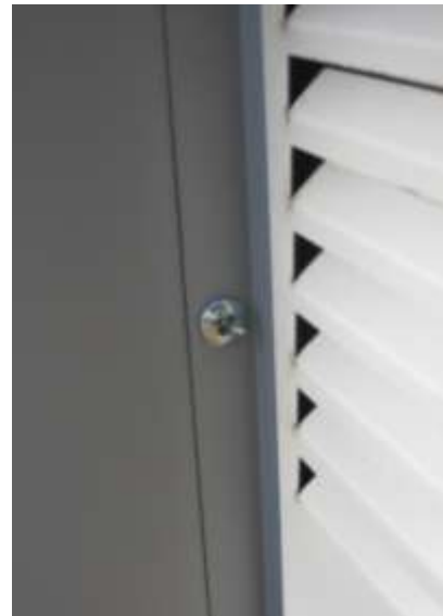
Step 23 screw in fixing bolts to connect heat pump module to storage tank
