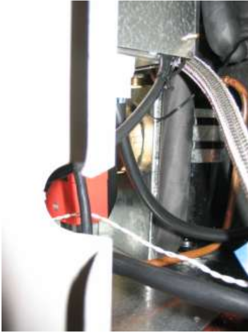
Step 18 remove the tab on the side of the electrical entry to the heat pump module
