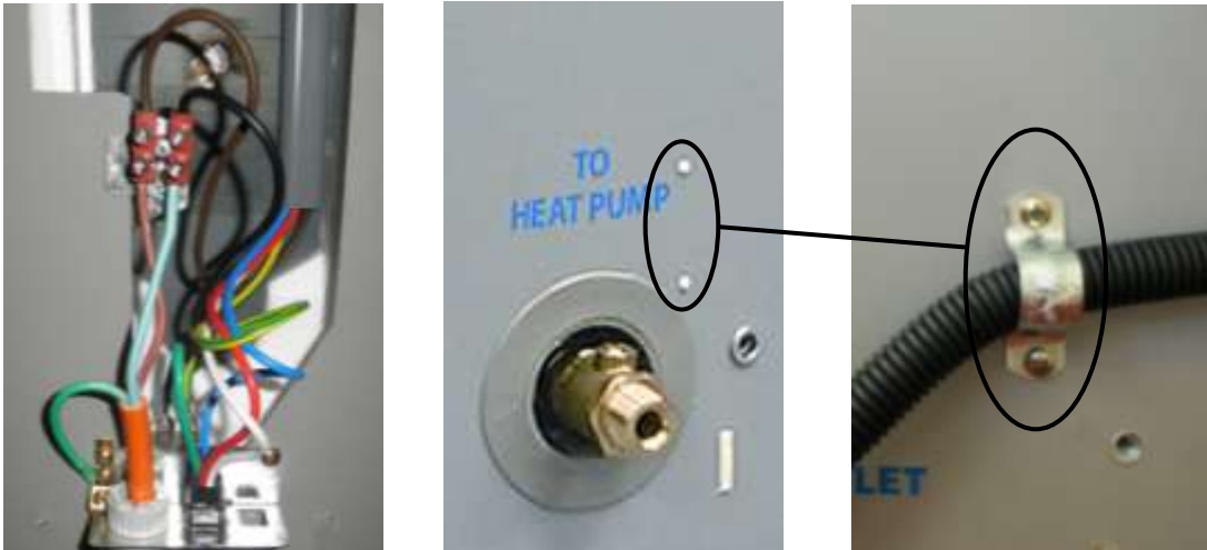
Step 4 connect wiring and secure conduit with saddle clamp
